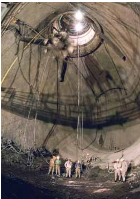
Fig. 3. Constructing a shaft inset on mine level 7 at Prosper-Haniel colliery.
