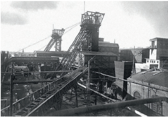
Fig. 2. Historical view on the colliery facility AV 1/2 of Auguste Victoria colliery.
