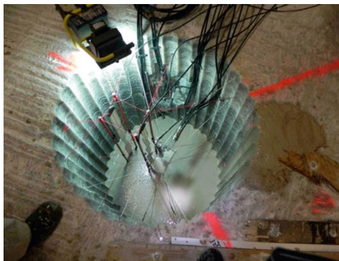
Fig. 4. Setting up the large-borehole trial to test formula-C 3 MgO concrete (3-1-8 binder phase)
