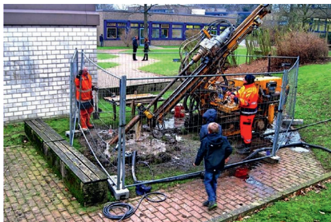
Fig. 5. Drilling operations during school hours.
