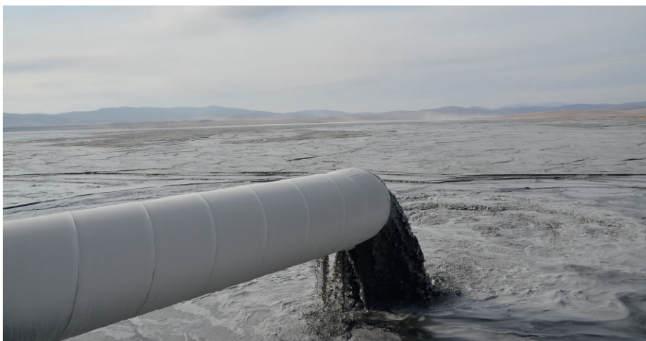
Fig. 3. Discharge of the residue from the ore processing facilities into the TSF.
