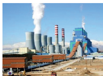
Fig. 4. The Soma Manisa lignite-fueled power station.
