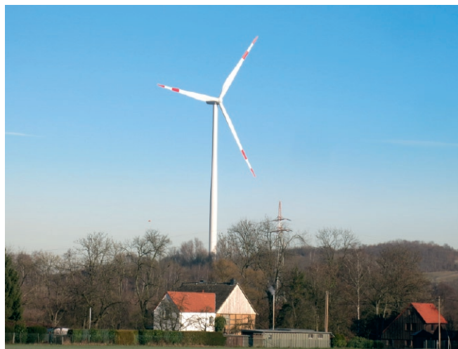
Fig. 2. RAG Montan Immobilien’s new wind turbine on the Elsa-Brändström-Strasse spoil tip in Lünen-Brambauer was commissioned in 2016.
