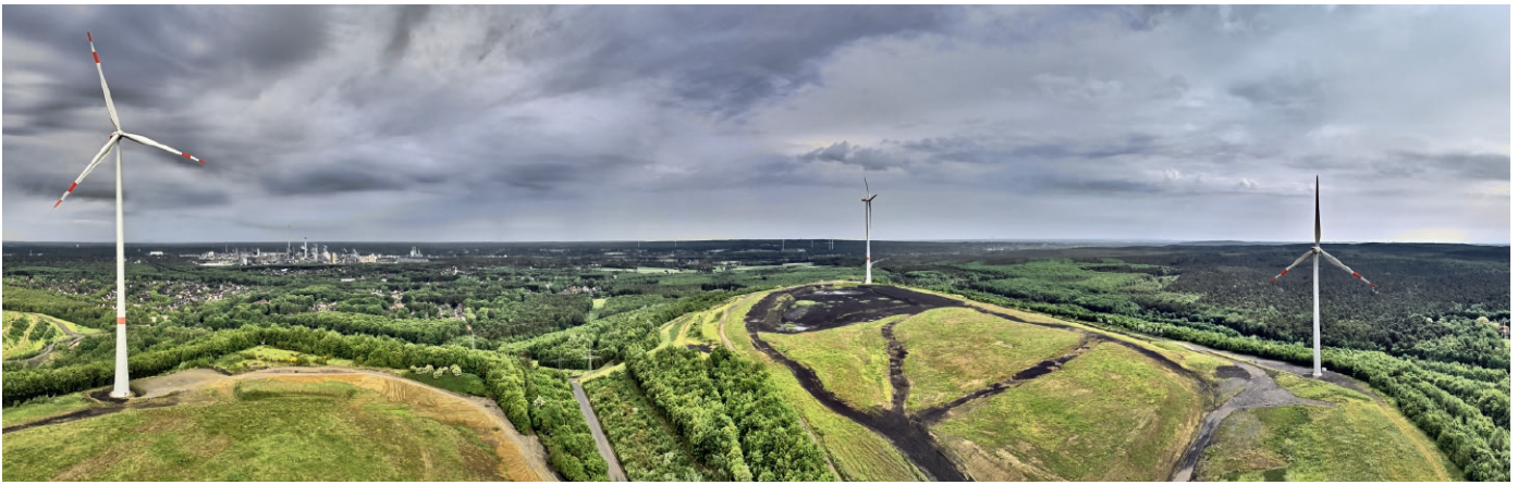
Fig. 1. Three wind energy plants on the Brinkfortsheide spoil tip in Marl are generating eco-friendly energy. All three wind turbines were built by Windkraft Brinkfortsheide GmbH, a subsidiary of the RAG Foundation and the RAG company.
