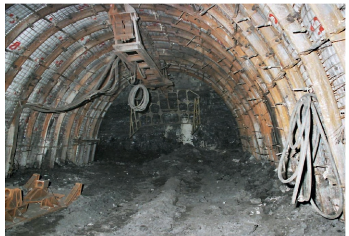
Fig. 13. Combined support type B.
