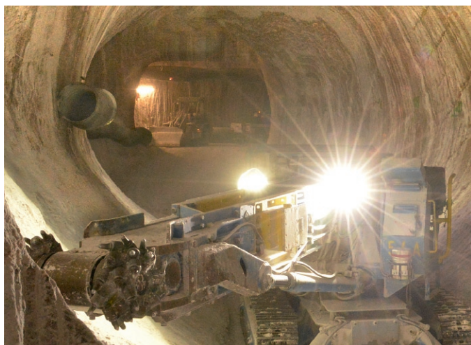
Fig. 7. Recutting at a planned barrier site.
