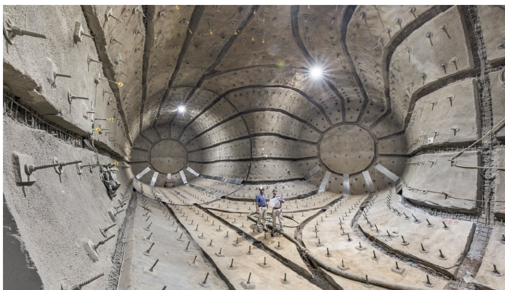
Fig. 3. Warehouse for liquid waste on the 850 m level (workshop for maintenance and repair work).
