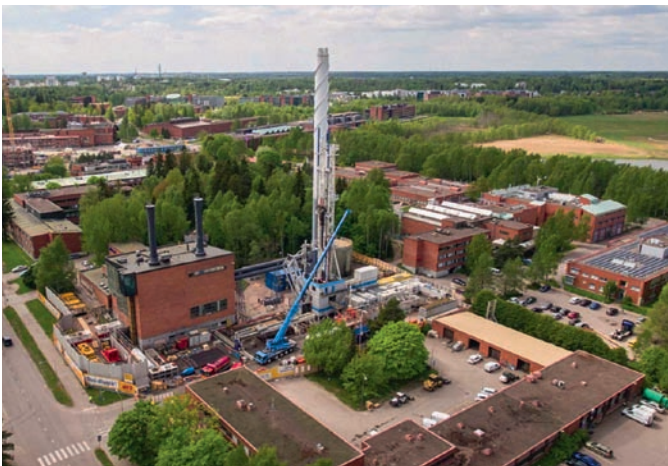
Fig. 2. Geothermal project in Helsinki.
