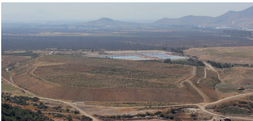
Fig. 5. Covered leaching heaps (leaching of oxidic ores) with collection ponds for the solution in the background. The facility is located west of Santiago de Chile (Lo Aguirre).
