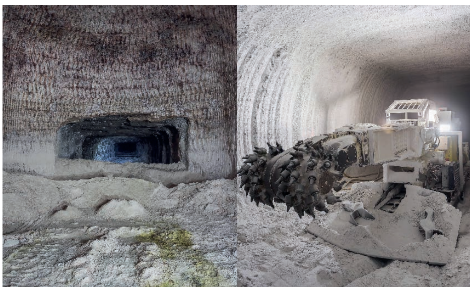
Fig. 2. Drift enlargement with a Roadheader AM 50.
