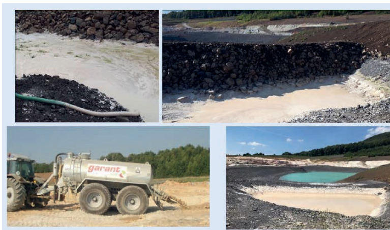
Fig. 4. R-basin with sludge collection basin.
