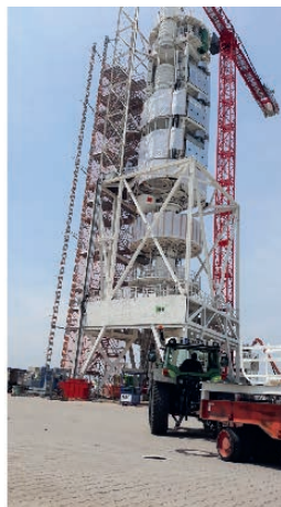
Fig. 8. Construction of two new potash shafts in Belarus.
