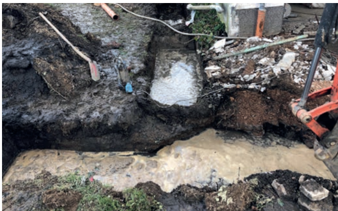
Fig. 2. Water level at the beginning of the investigation.
