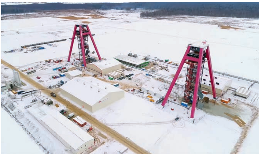
Fig. 1. View of the construction site in January 2019.
