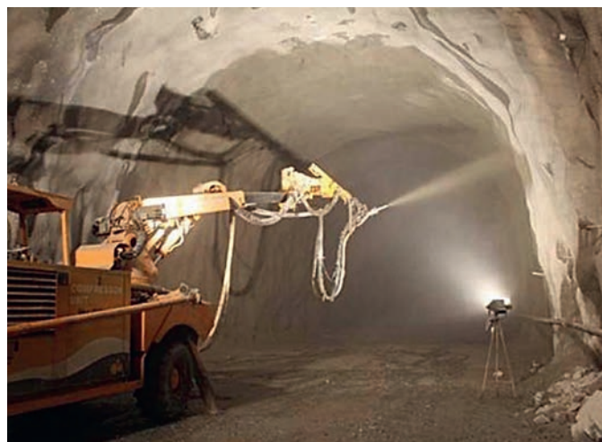
Fig. 2. Shotcrete work in the tunnel.
