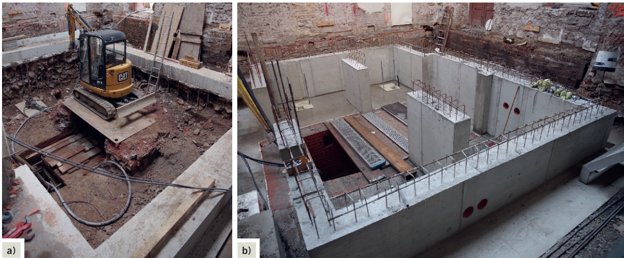
Fig. 4. Excavation pit (a) for the new pit frame foundation (b).
