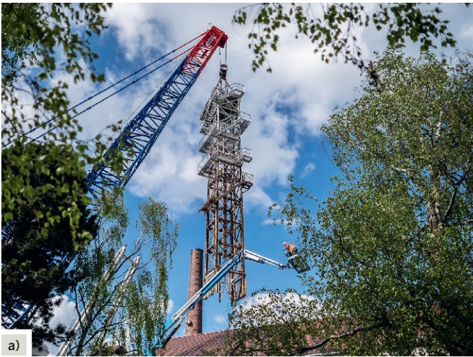
Fig. 3. The guide frame (a) and the diagonal brace (b) were lifted out of the shaft house.
