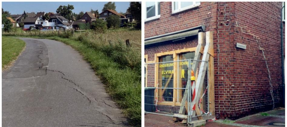
Fig. 1. Earth tread formation in the Erkelenz district between two localities (left) and on a building (right).
