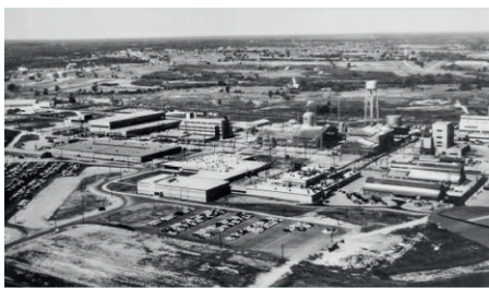
Weldon Spring, MO Uranium Feed Materials Plant, ca. 1957.
